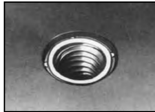
5. Installed Insert
